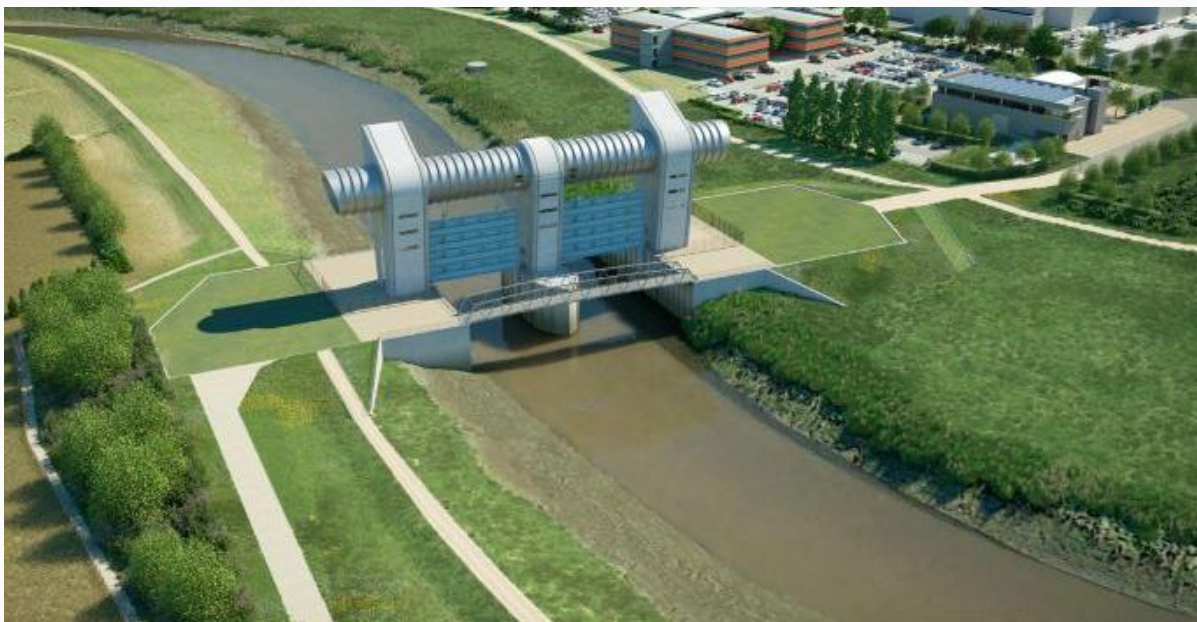
Bridgwater Tidal Barrier
